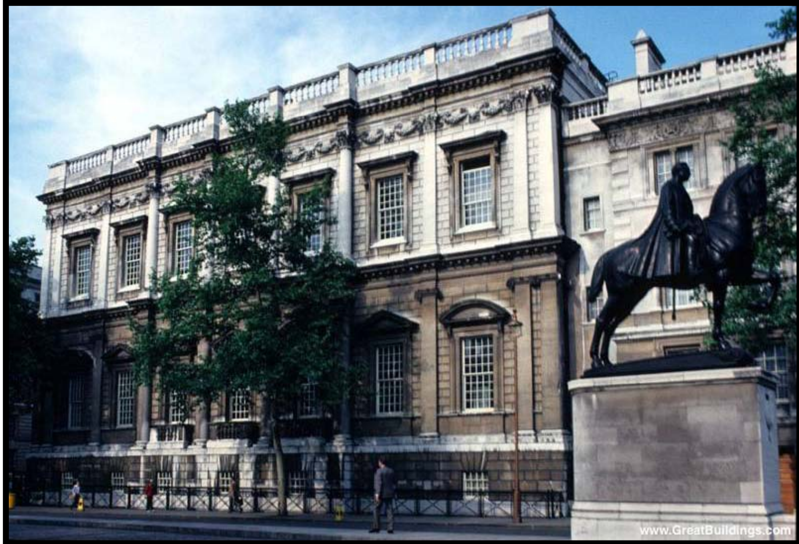
JONES, Inego Banqueting Hall Whitehall
